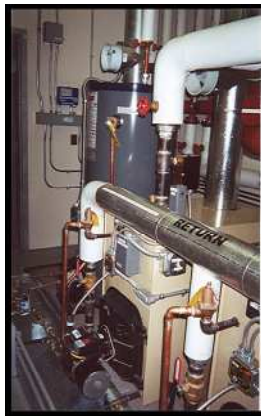
NEW BOILERS & HW HEATER
